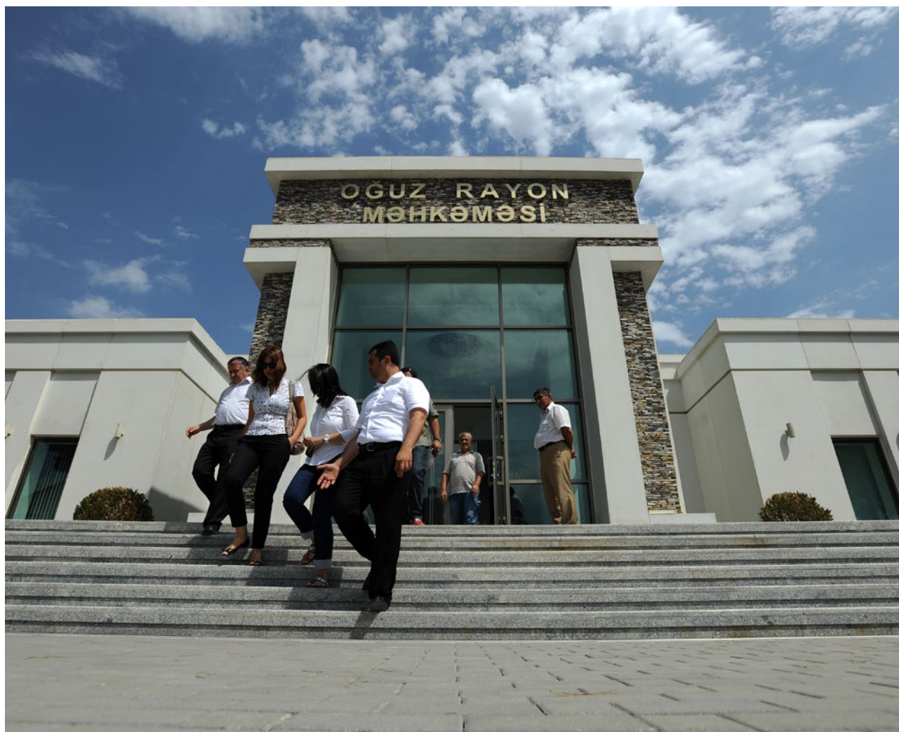
New courthouses in Azerbaijan financed by the World Bank aim to make the judiciary process faster and more efficient. Photo: © Allison Kwesell / World Bank.
